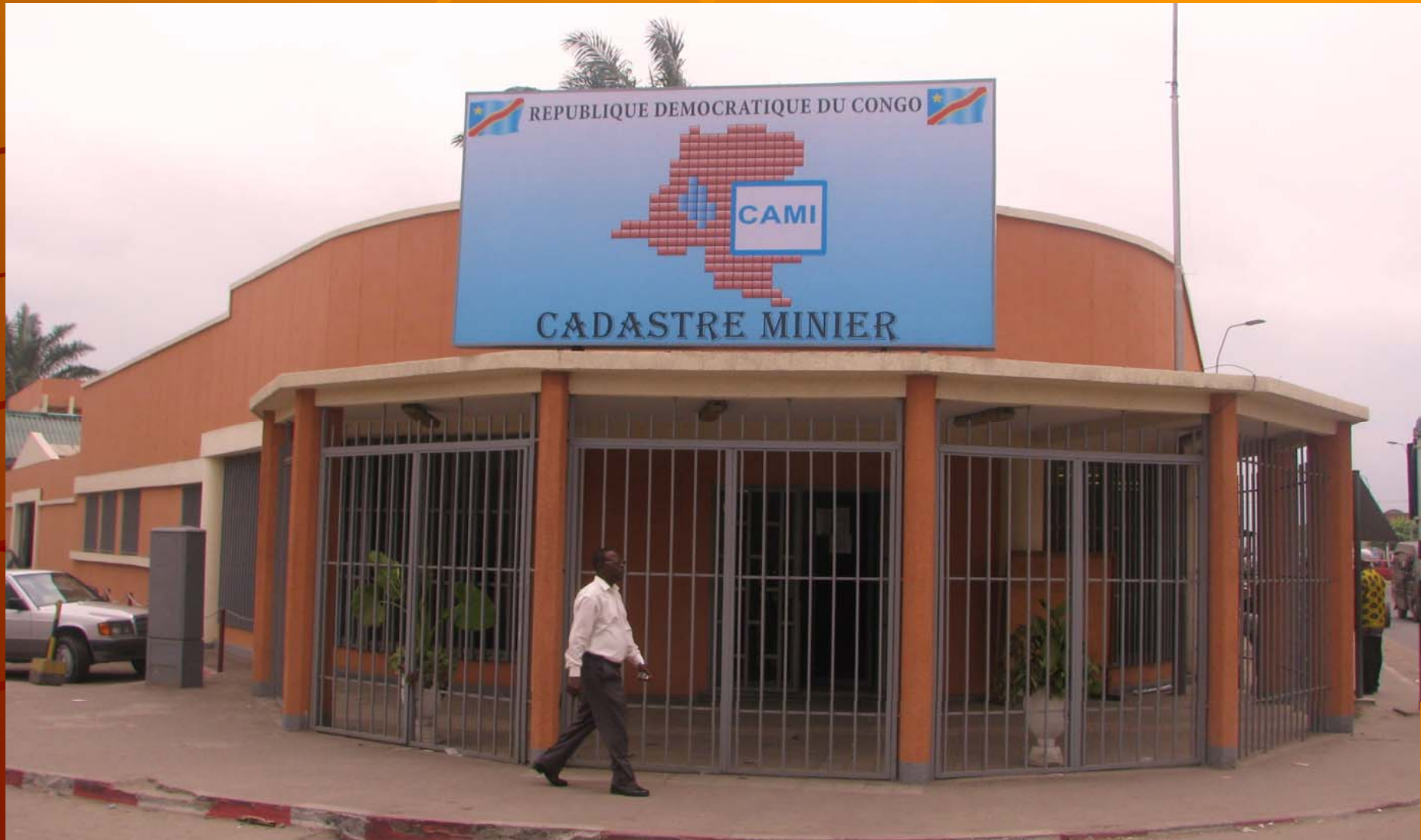
THE CAMI MAIN OFFICE
